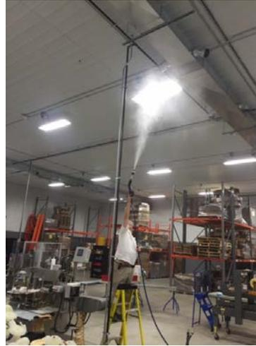
A Manufacturing Company who makes products utilizing the process of boiling, which produces steam, is at risk for contaminating their finished products with mold, mildew, algae and fungi. Even in a metal building, the collection of steam (vapor-moisture) on surfaces can present a problem with mold. The surfaces that collect the moisture cannot always be dried; therefore, a process to rectify the situation needs to be employed. Bactronix provides the perfect solution
